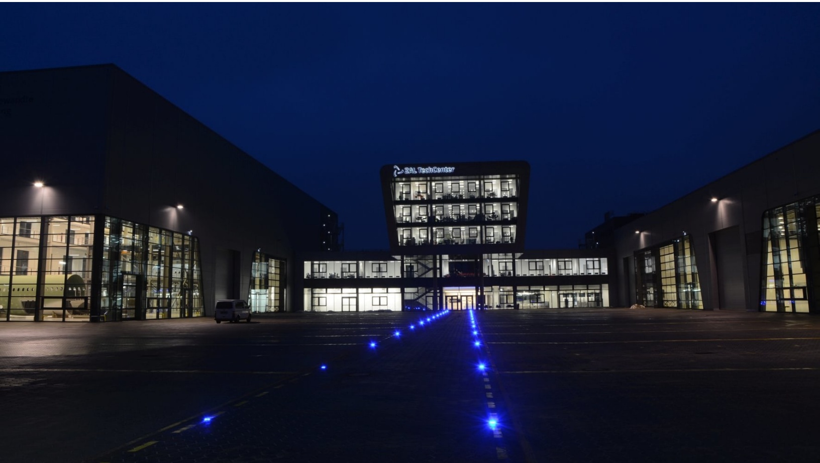
ZAL TechCenter in Hamburg (Copyright: Paul Milbrod, Ed. Züblin AG)
